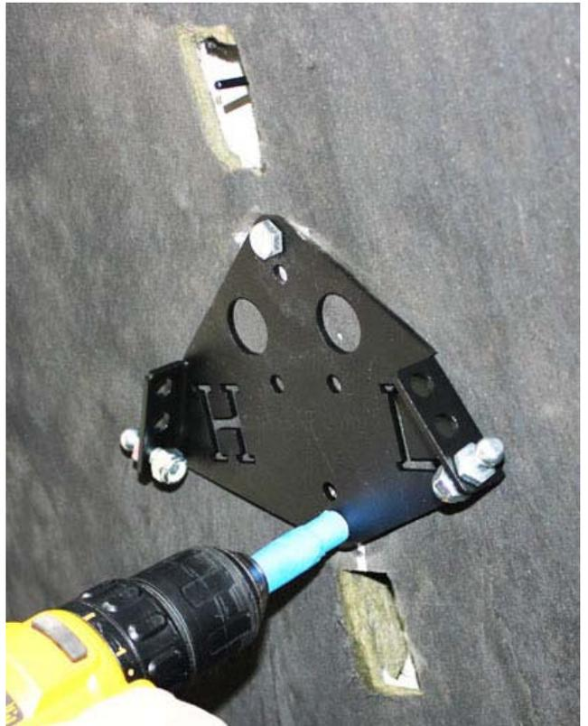
Drill 2<sup>nd</sup> hole, using bracket as a template, then install lower bolt as you did the upper one.
